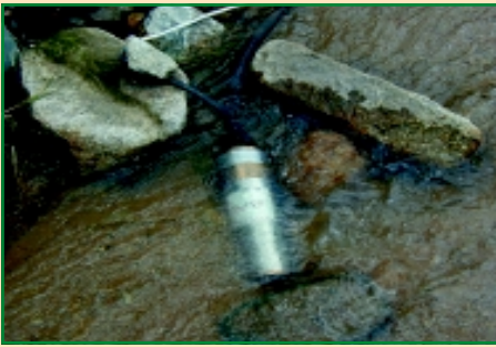
Figure 5: Solar powered water pump
