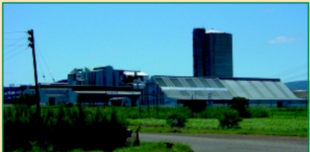
Figure 23: Ubombo Sugar Mill, Big Bend, which generates heat and power from bagasse
