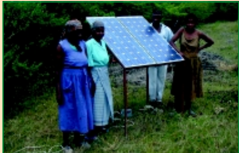
Figure 6: Solar panels to power water pump
